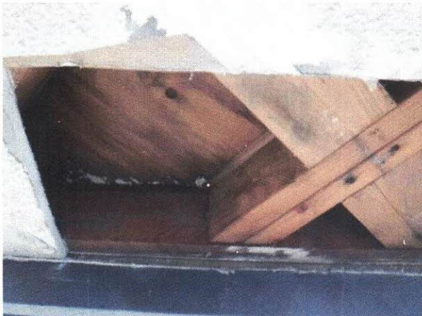
Photo 26: Exploratory opening at soffit. (Unit 302)
