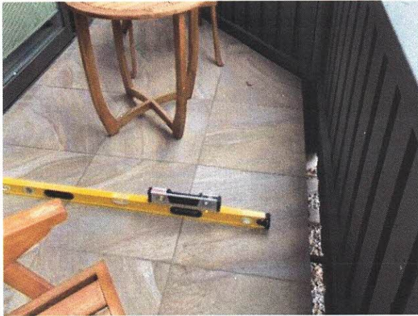
Photo 6: Tile installed over concrete topping slab.
