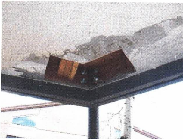
Photo 32: Exploratory opening at soffit. (Unit 201)
