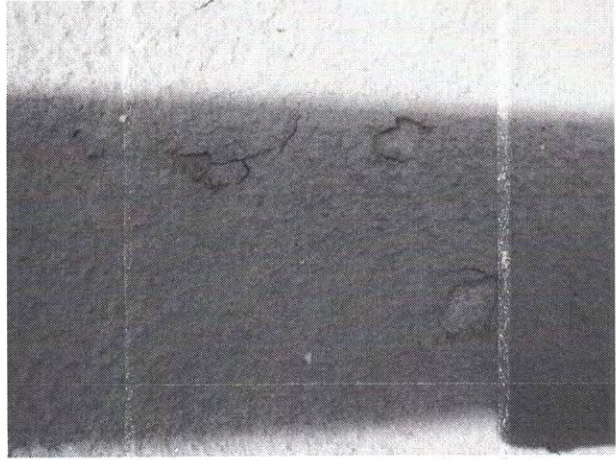
Photo 7: Minor deterioration of wood trim adjacent to balcony. Note the balcony at this location has been coated.
